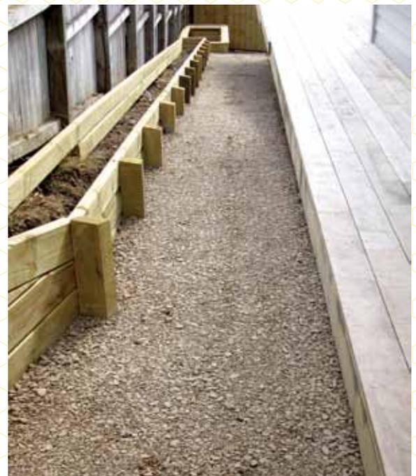
Step 5: A topping layer is recommended above the top of the JakMatEnviro, compaction is done with a plate compactor ensuring a sound and professional finish
