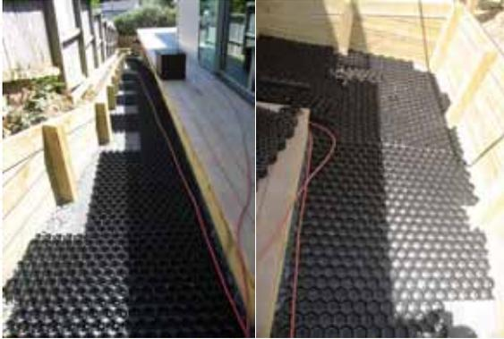
Step 1: Ground prepared and leveled with Gap7 aggregate used as bedding material
